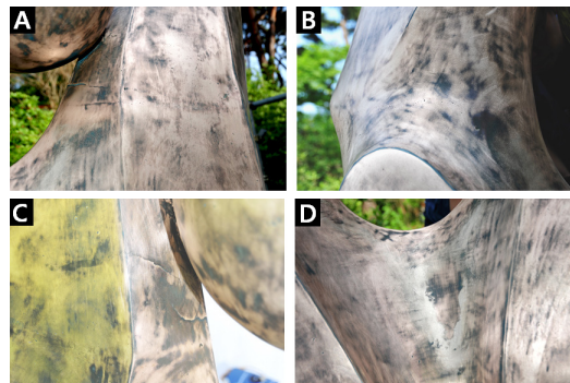
Figure 2. After polishing the surface defects. (A), (B) Welding blowholes, (C) Welding crack, (D) Light stain(Segregation).
